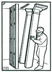
Locate column cover half as identified by the larger vertical flange and position over scribed circular line on floor.
