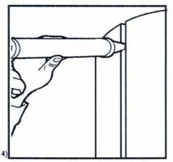
Using a low modulus, paintable caulking, caulk all seams including horizontal reveals at floor and ceiling.
