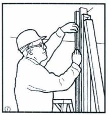
Scribe line on structural column at height "Y" as measured in step (6).
